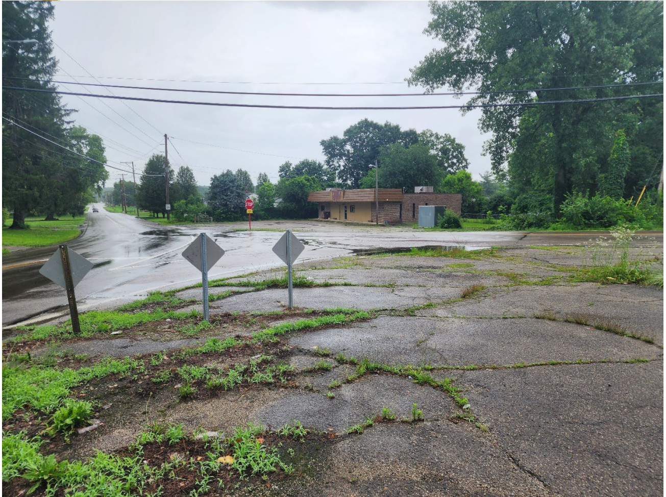
6000 Philadelphia Drive, looking from 5990 Markey Road across the intersection of Markey & Philadelphia
